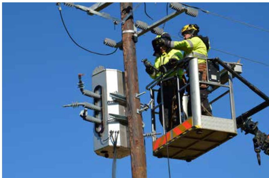
The monitoring and control cabinet that is sold with the Auguste solution is used to remotely or locally monitor and control the Auguste switch, according to the customer's requirements.
