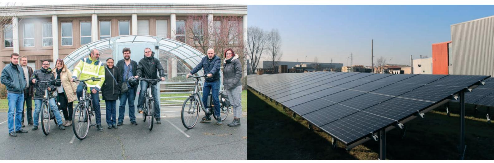
At left: Electric bicycles and their sheltered charging station. At right: Five hundred solar panels occupy 2,000 square meters, covering roughly 30 percent of the factory's needs for electricity.
