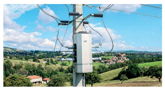
Auguste switch disconnectors isolate automatically a faulty part of a network and thus allows to re-energize all the remaining healthy network
